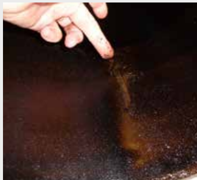
Deposits in tank
