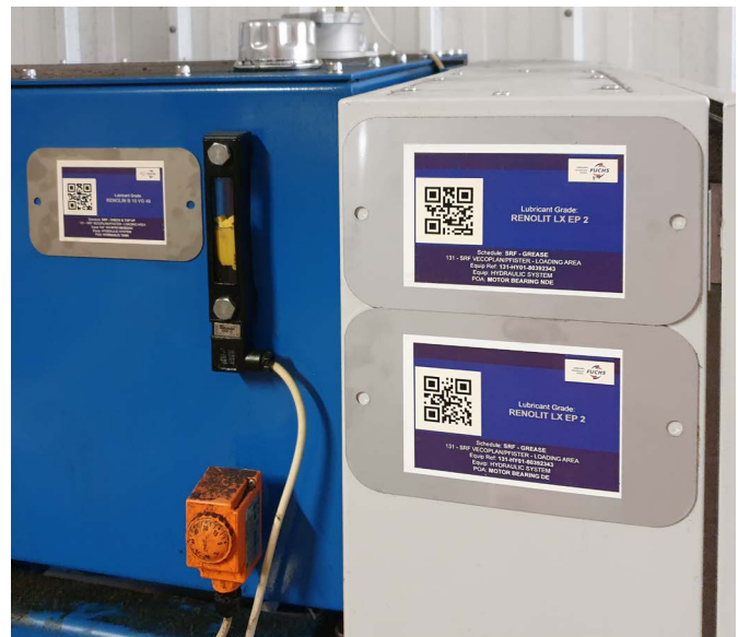
FluidsConnect uses QR code scanners to record machine specific content.
