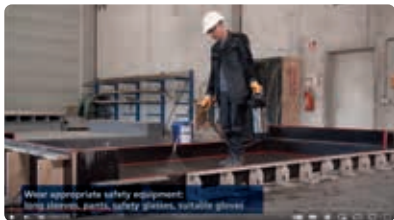
Application of concrete release agents
